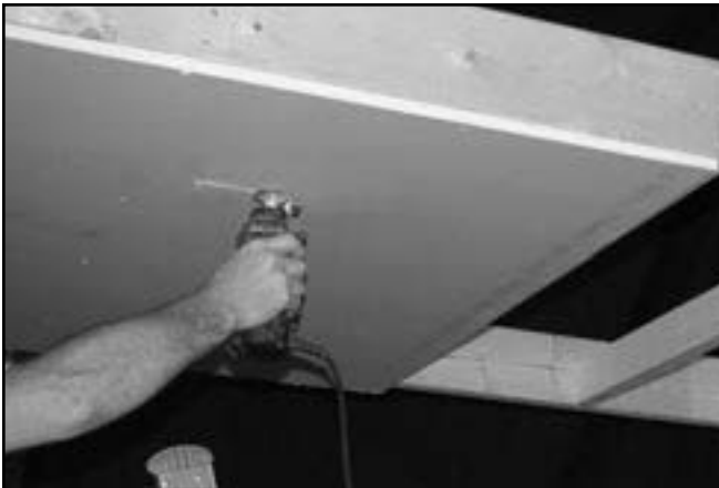
Figure 5: Cutting drywall using the Rotozip™.
